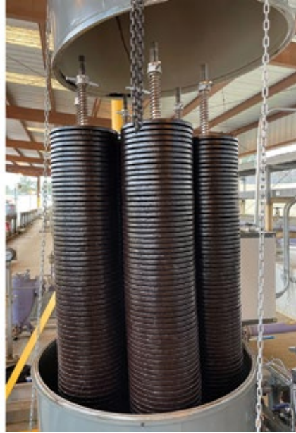
8. Filter elements capable of removing contaminants and water from distillate oil are being installed at left. Effectiveness of those filter elements in removing solid contaminants that could impede reliable operation of a standby fuel system is in evidence at right; water is removed in the second stage of the two-stage system. For the case illustrated, more than 340 lb of contaminants were removed by one set of depth-filter elements in four weeks
