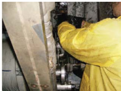
F. Protective clothing is required by hydrolaze technicians
